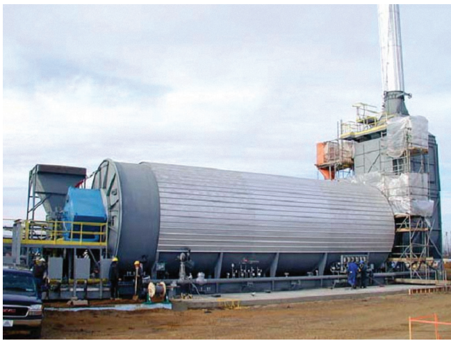
OTSG unit with QLN burner.
