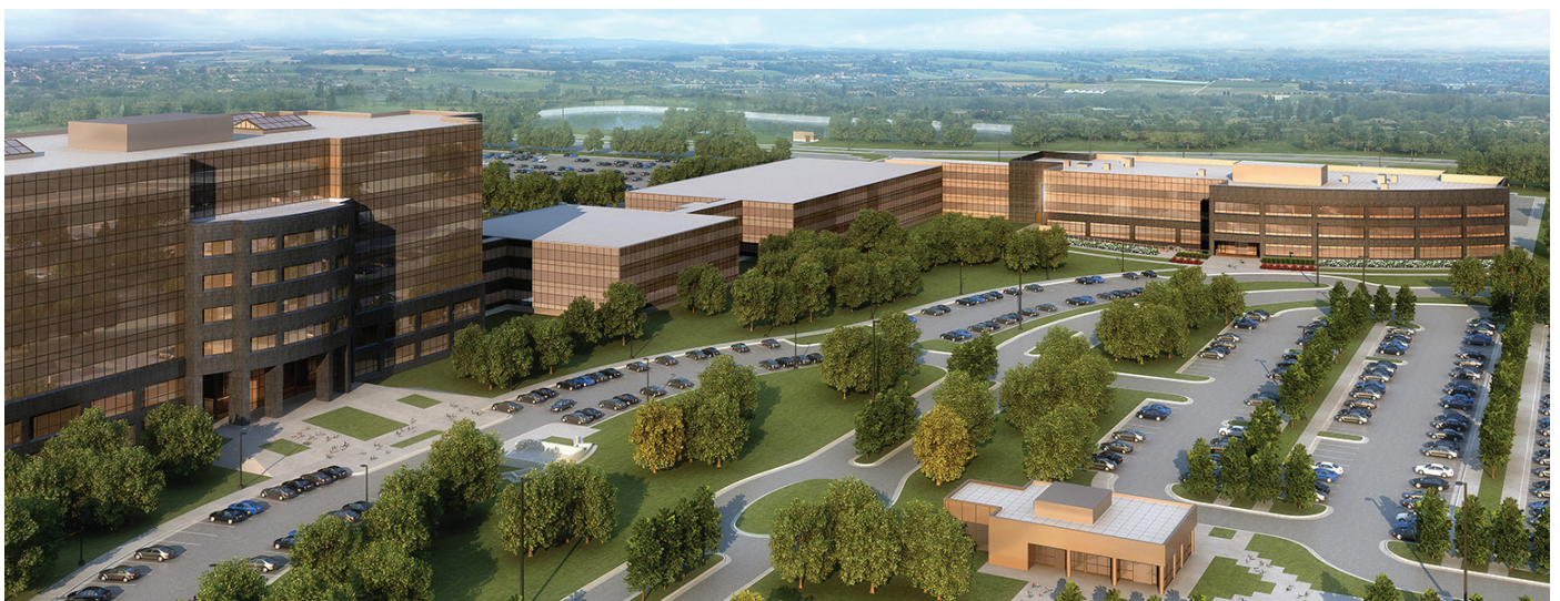
KOCH INDUSTRIES CORPORATE HEADQUARTERS, WICHITA, KANSAS, USA. ALSO LOCATION OF KOCH-GLITSCH WORLDWIDE HEADQUARTERS.
