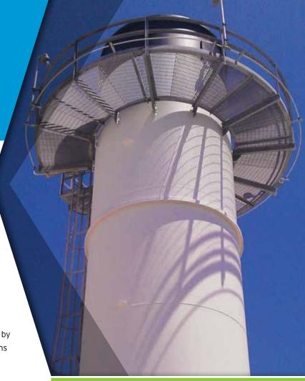
Our NOxSTAR Vapor Combustion System provides up to 99.99% destruction efficiency with less than 0.02 lbs NOx/MMBtu and less than 0.015 lbs CO/MMBtu.
