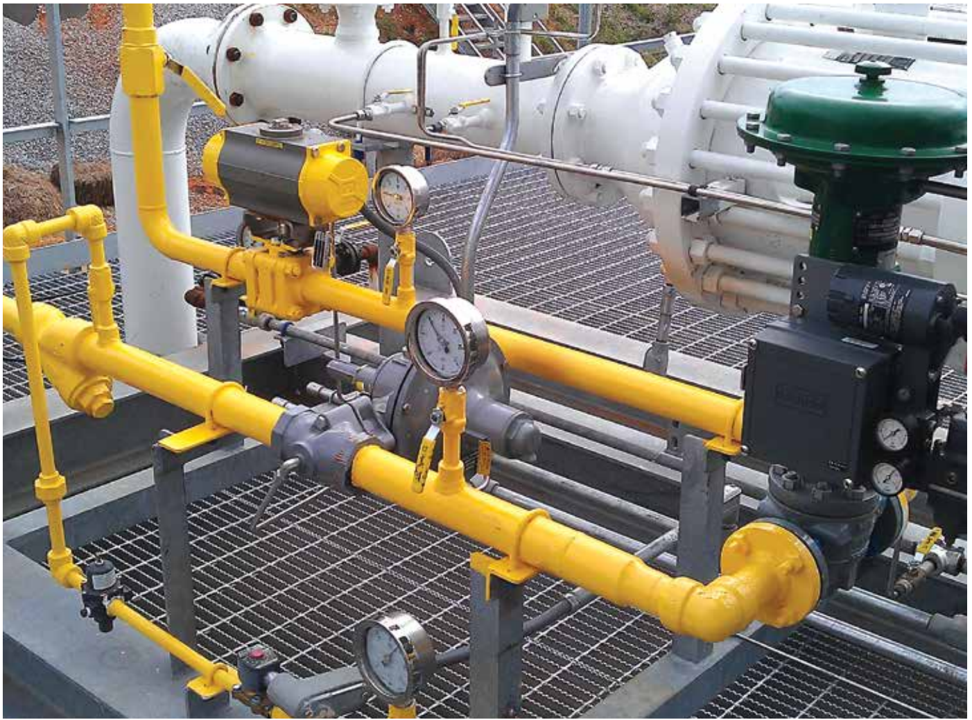
VAPOR ENRICHMENT TRAIN ON A DOCK SAFETY UNIT
