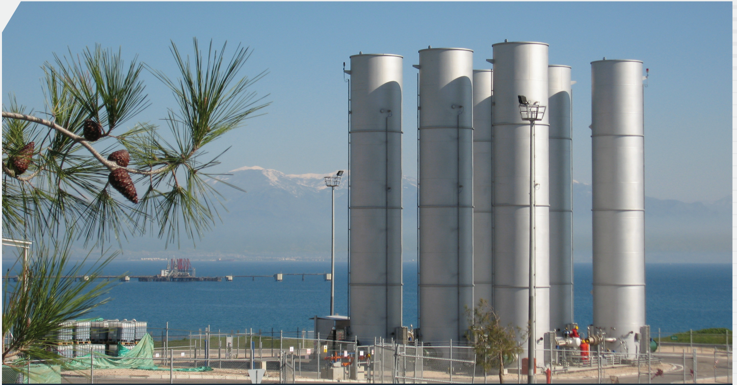
Multi-Stack Marine Vapor Combustion System
