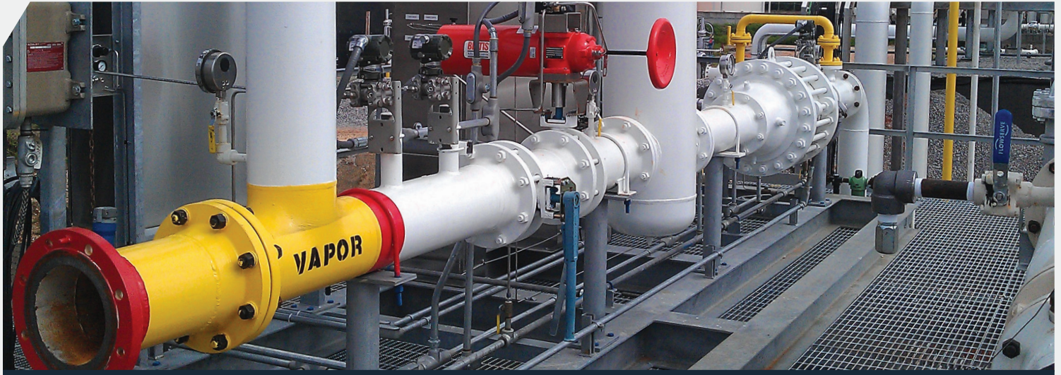
Dock Safety Unit
