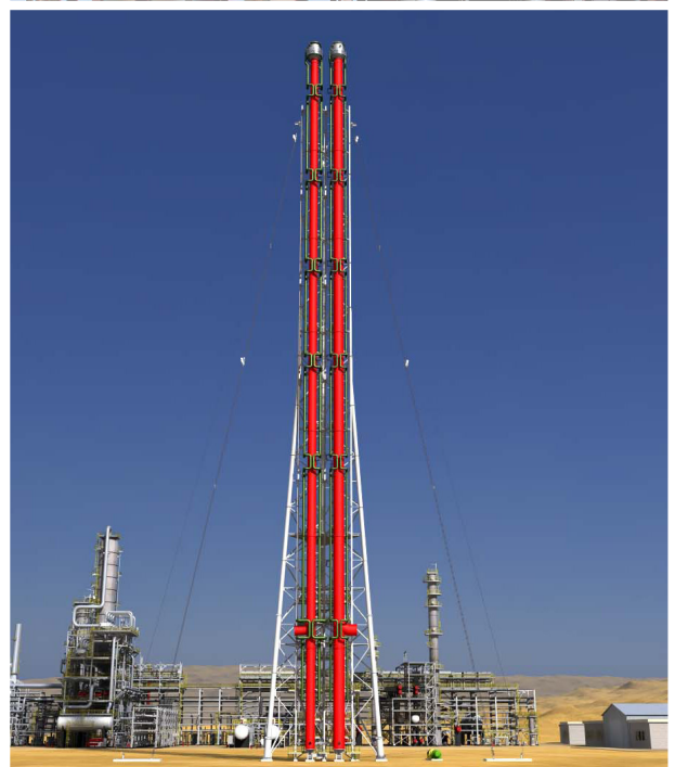
Demountable flares allow flare tip replacement with adjacent flares in service.
