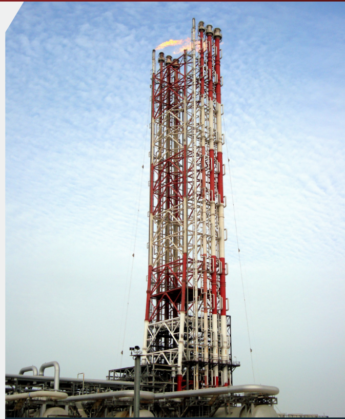
Multi-Flare Tip Demountable Flare Structure
