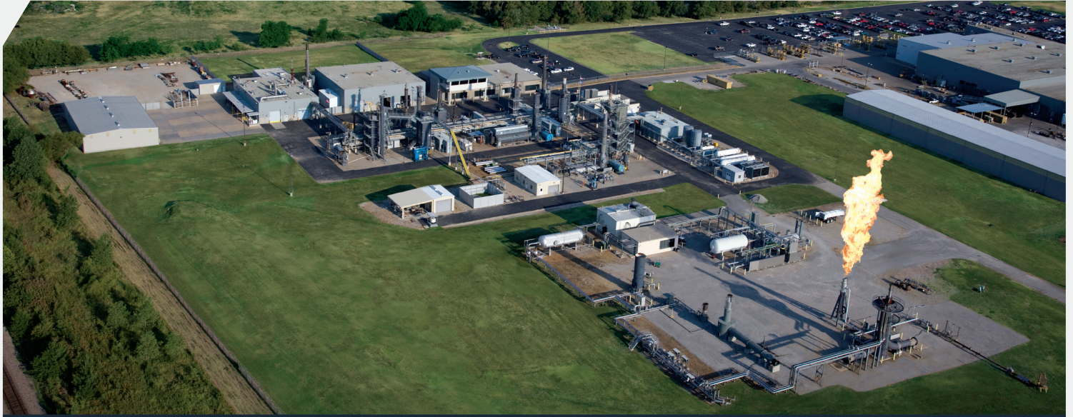
Research And Development Test Center
