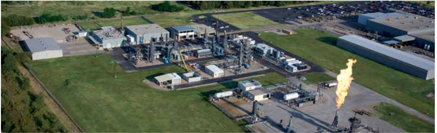
RESEARCH AND DEVELOPMENT TEST CENTER
