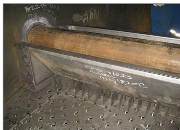
Figure 4 New liquid feed distributor
