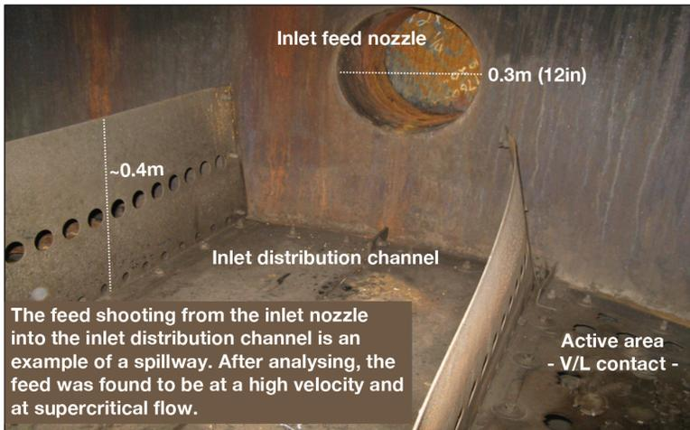
Figure 2 Existing liquid feed arrangement
