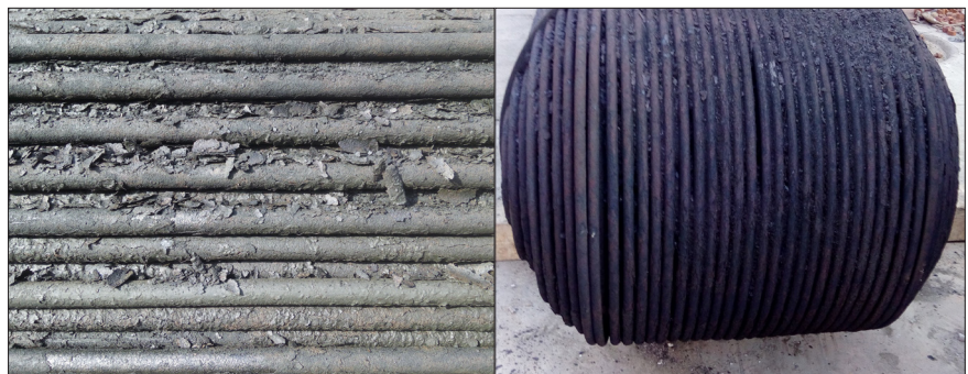
Figure 6 Fouled debutaniser reboiler tubes
