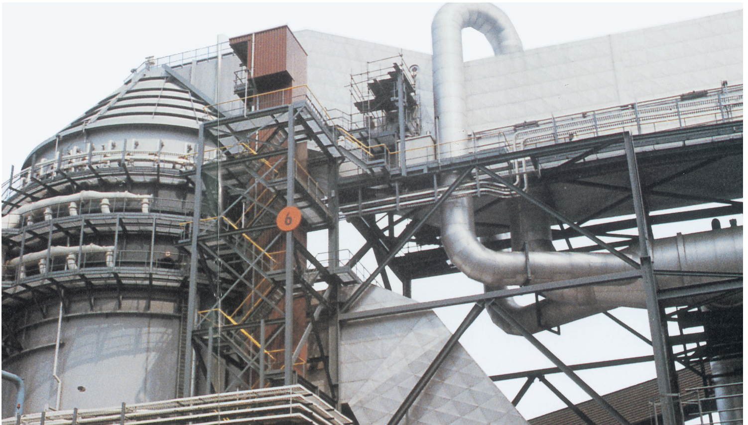
Side view of a two stage FLEXICHEVRON® and Washing System in a vertical tower.
